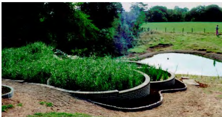
A vertical flow system designed by Burka at Oakland Park, Gloucestershire, in its first summer of operation (Burka & Lawrence 1990). The mature system is shown on page 1 of Part 1.
