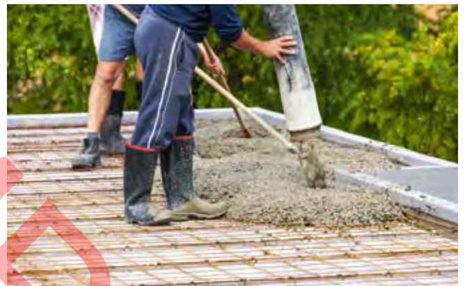
Figure 1: A domestic reinforced in situ concrete floor slab being poured
