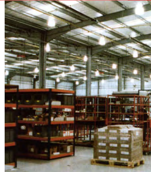
Lighting scheme in a new factory unit, comprising metal halide lamps controlled in zones by manual switching. It uses high efficiency modern components and exploits natural and reflected light potential
