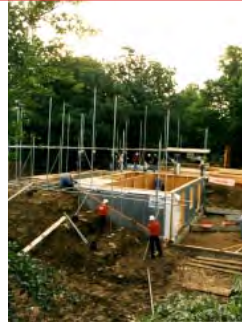
Figure 1 Semi-basement under construction for the BRE Integer House
