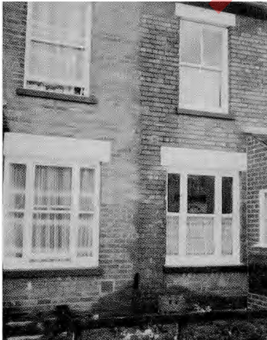
Repointing has restored weathertightness to the house on the left
