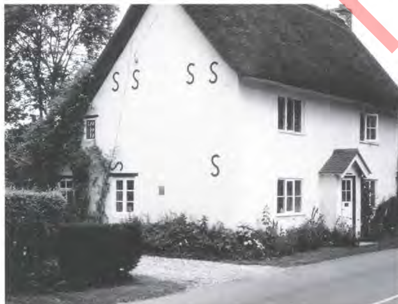
Figure 1 Traditional cottage with remedial through-tied gable walls
